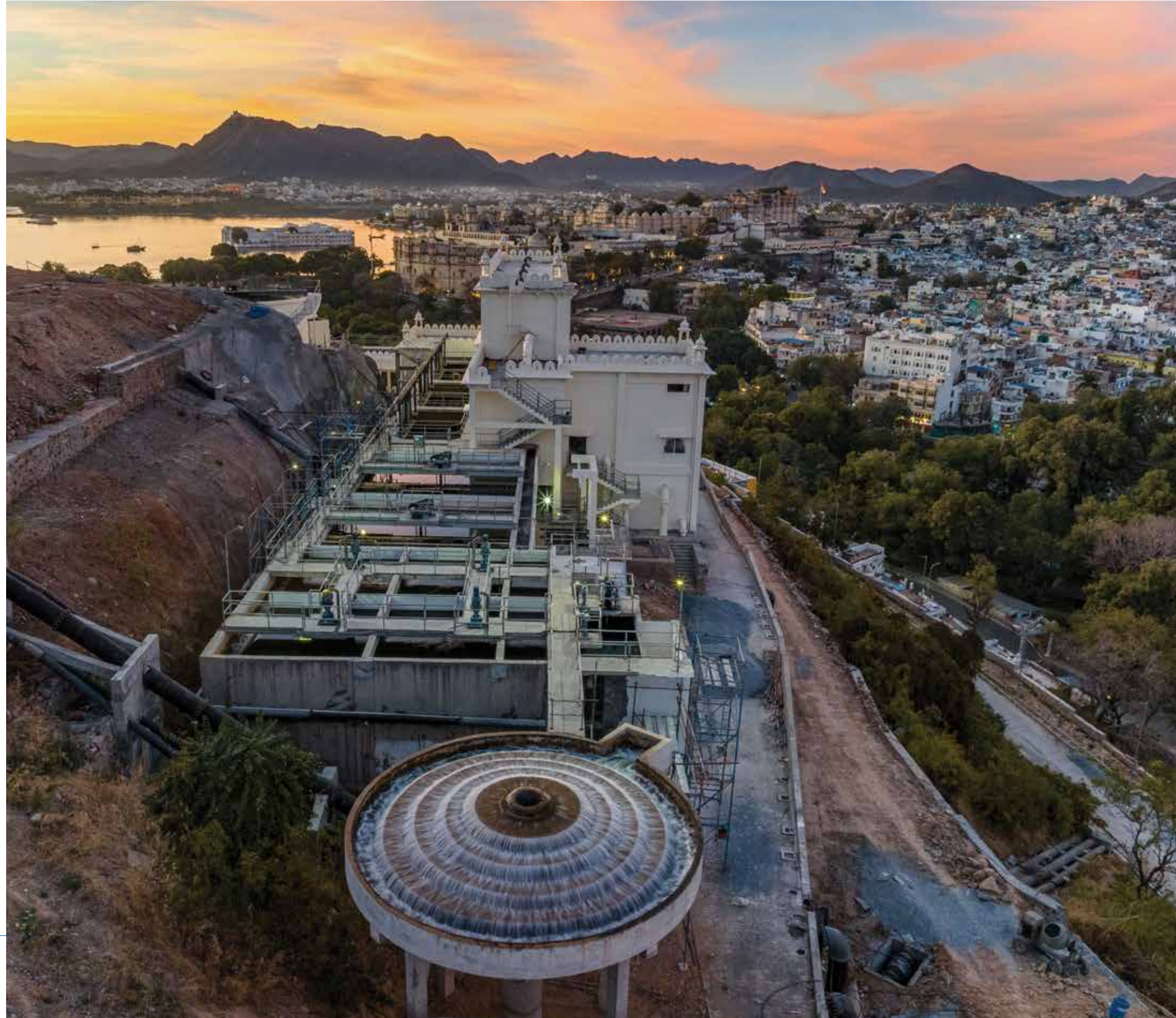
Left : Aerial view of different treatment units of WTP
