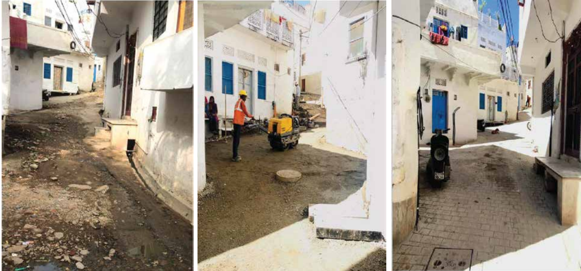
Left : Before construction of sewerage network
