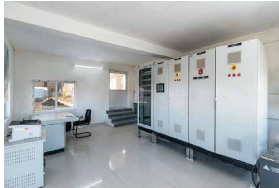
Top : 23.47 MLD Water Treatment Plant Bottom Left : Filter Back wash Pipeline Bottom Right : Machine Room , WTP Right Page : Gravity Suldge Thickener
