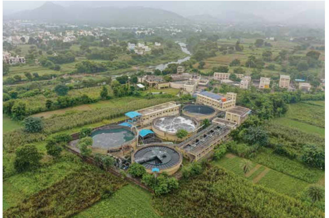
Left : Main Purification Tank
