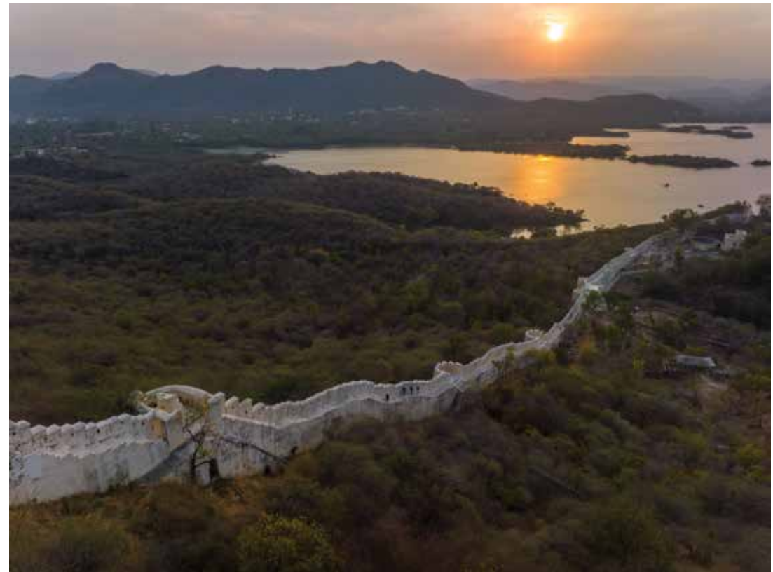
Left : Fort Wall leading to Karni Mata Temple Right : View of Fort Wall & Lake Pichola from Karni Mata Temple Right Page : Fort Wall from Chandpole to Swaroop Sagar
