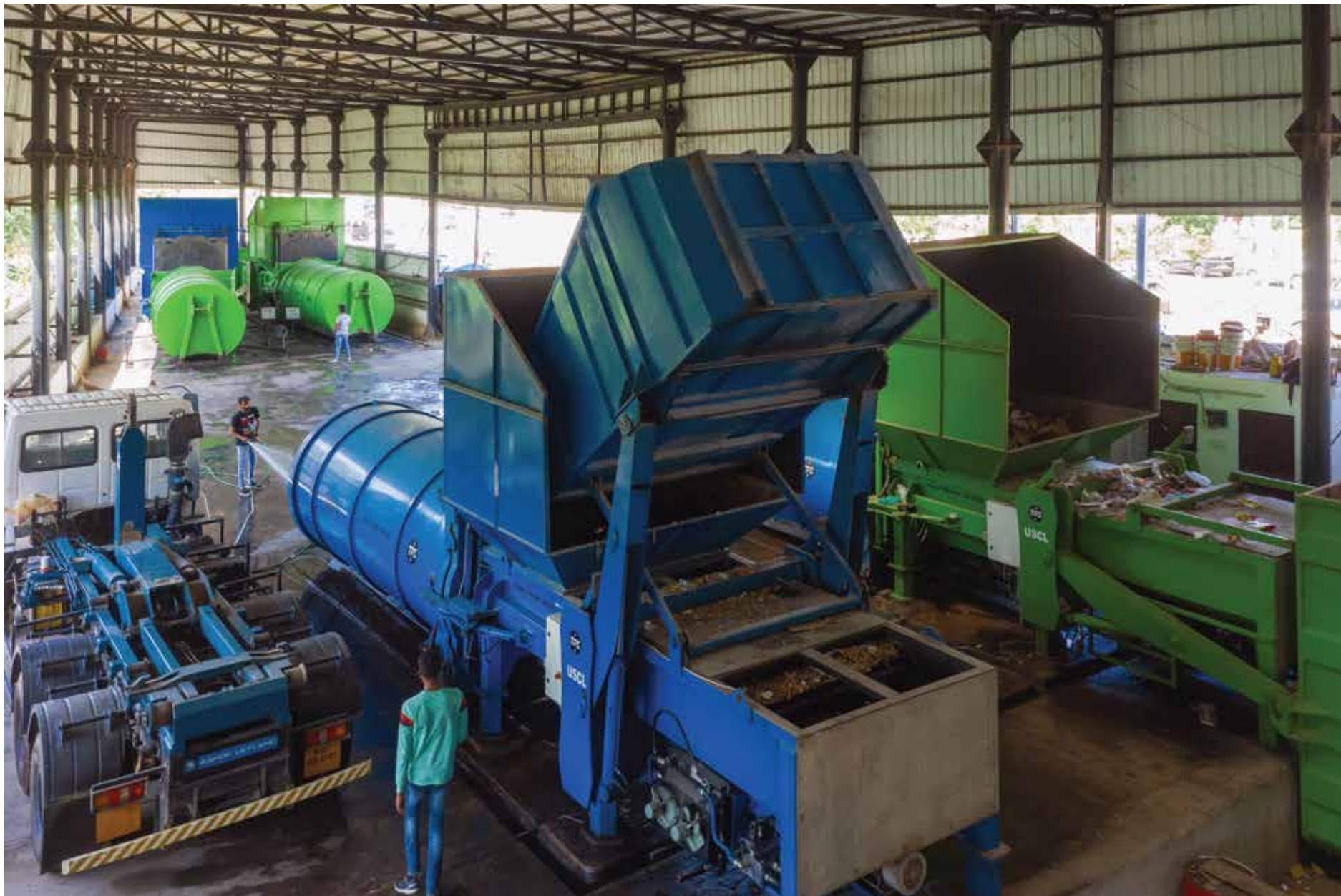
Above : Transfer Station, Kumharo ka bhatta
